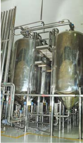
The basic shampoo production process involves batches of raw materials (chemicals) prepared, weighed, and then aggregated in large mixing tanks.
